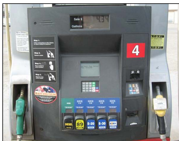
Figure 8. Station #14 offered higher ethanol blends from the same hose as E10
