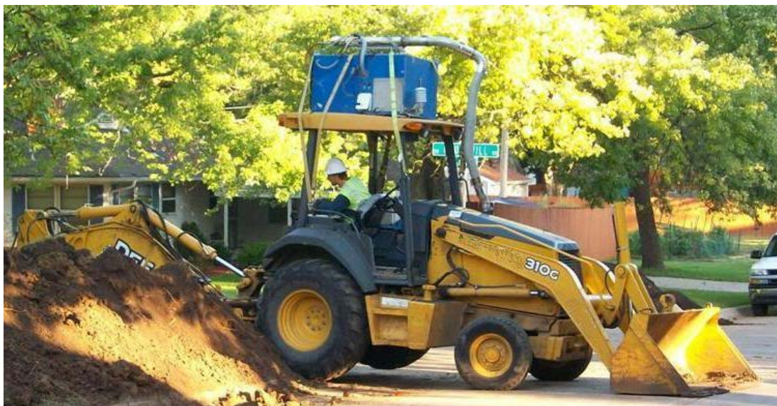
Figure 7.3-3 Backhoe Loader with Metal Tubing Installed
