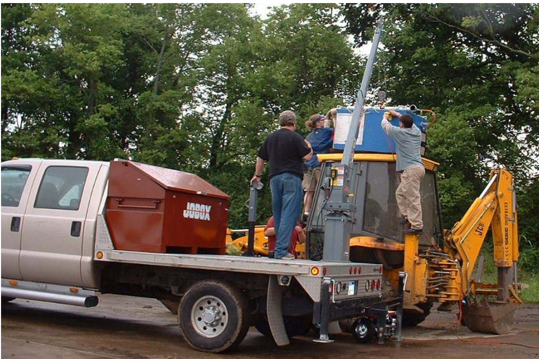
Figure 3.4-2 Installation of PEMS Rack Using Truck-Mounted Boom
