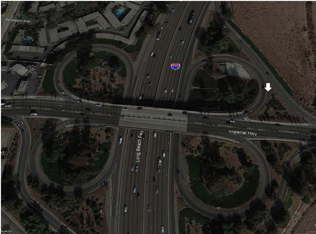
Figure 6. Satellite image showing the location of the Lynwood I-710 emissions sampling site (arrow) located on the off-ramp from northbound I-710 to westbound Imperial Hwy. in Lynwood, CA.
