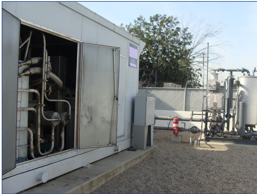
Figure E.4 Drier System and Compressor Skid at Station W1
