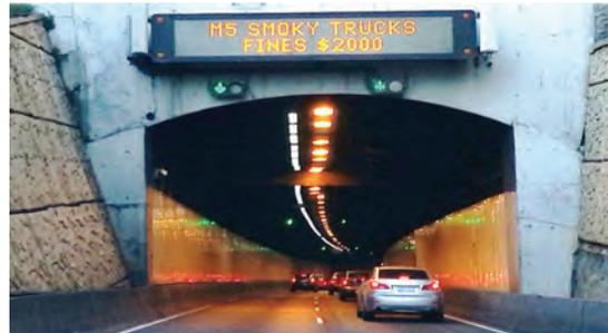
Figure 6. (bottom) Opacity sensors and video cameras identify high-emitting vehicles in a tunnel in Australia.
